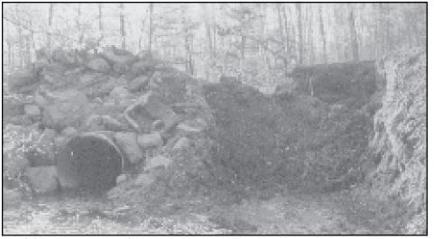
UNCOVERED BRIDGE - While excavating to install a second culvert under Bower Road, the town crew discovered the remains of a 12 foot wide concrete box bridge that had been buried when the original road was improved long before highway department records were kept. No treasure or skeletons were found.
