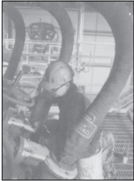
**UPKEEP** - Mechanic Mark Fenner maintains the primary hydrocyclone. After the sulfur dioxide that's been scrubbed from the flue is processed into a gypsum slurry, this machine separates the slurry so it can be dried into useful gypsum.
