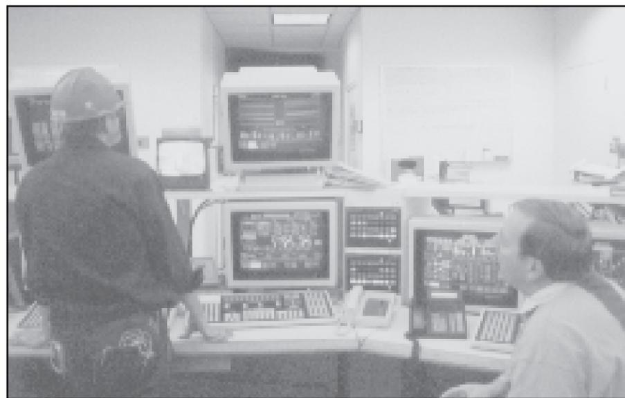
**COMPUTER HORSE SHOE** - Shift Supervisor Ron Marshall and Unit Two Control Operator Ron Baker monitor the Flue Gas Desulfurization unit that "scrubs" 98 percent of the sulfur dioxide (SO<sub>2</sub>) from stack emissions. Not only does this reduce acid rain, but the snared SO<sub>2</sub> is transformed from a noxious gas into gypsum which is sold for use in sheetrock.
